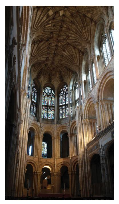
Figure 1: The presbytery of Norwich Cathedral. Although the current clerestory was remodelled in the 15th century, the disjuncture between Romanesque and gothic architecture above the first floor is a direct result of damage caused on St Maur(us)'s Day 1362. (Photograph by the author).
